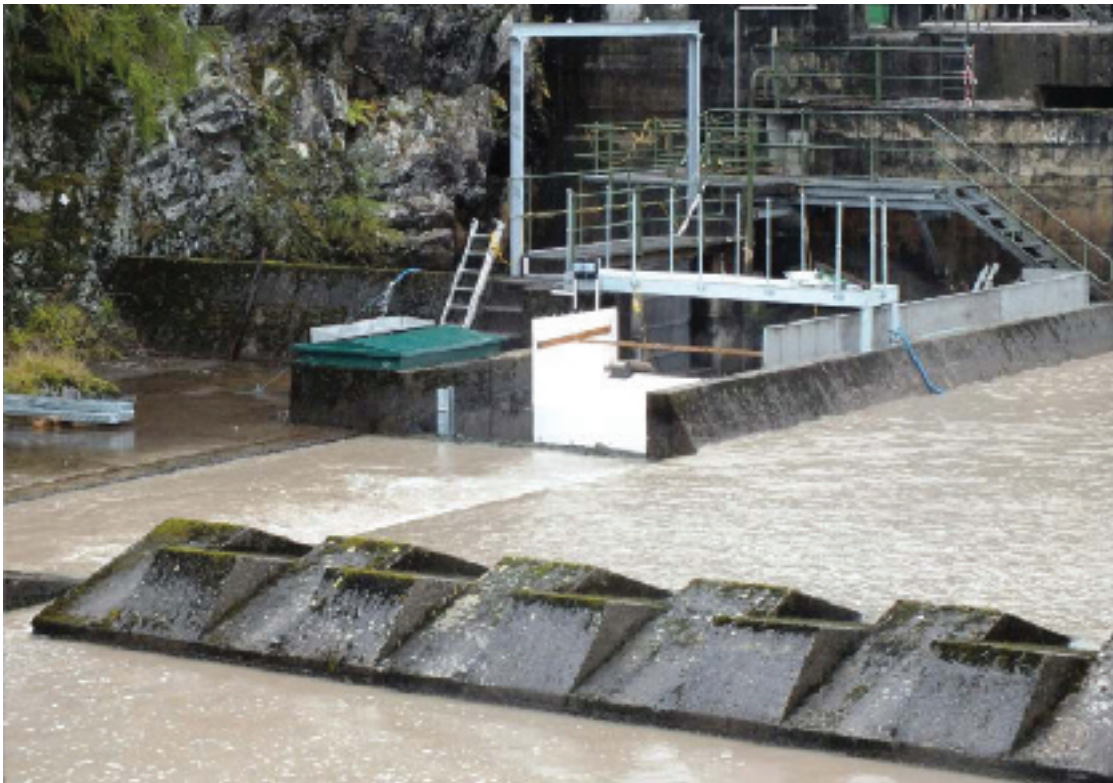
RTA installed a resistivity counter immediately below the fish pass at Spey Dam in 2012 to try to monitor the numbers of adult fish ascending and descending the fish pass. The coloured water was due to a significant landslide in to the Markie Burn, which enters the Spey immediately above the Dam.
