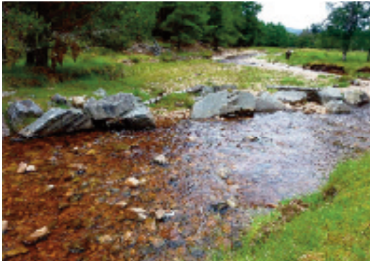
Before: rock armouring in place.
