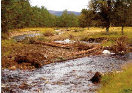
After: rock armour removed and replaced with wooded debris.
