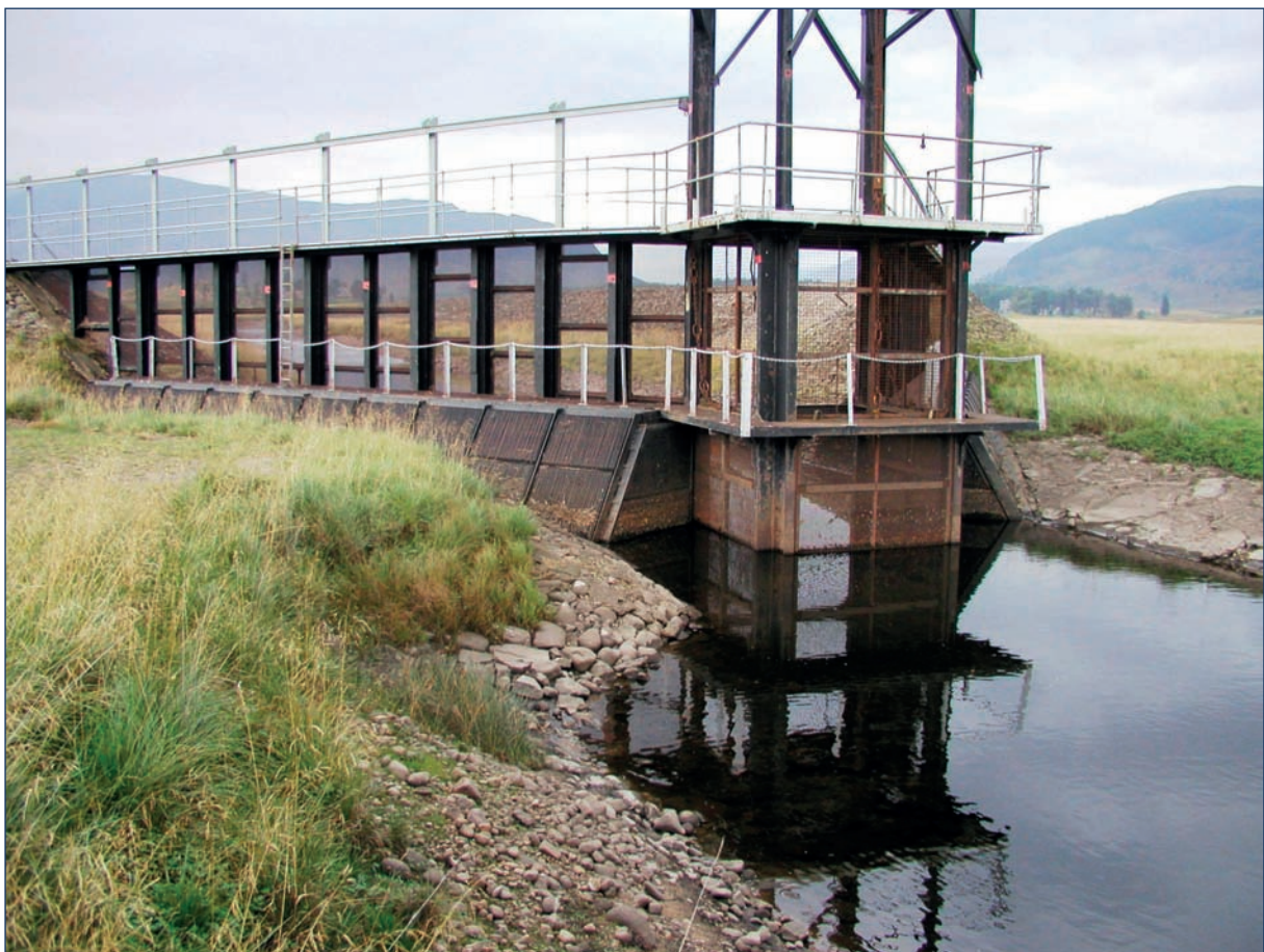
The off-take above Spey Dam, through which water is diverted to Loch Laggan. The Board is concerned about the efficacy of the screens and off-take in preventing juvenile fish from exiting the River Spey and its catchment and gaining access to Loch Laggan. (Photo: Roger Knight).
