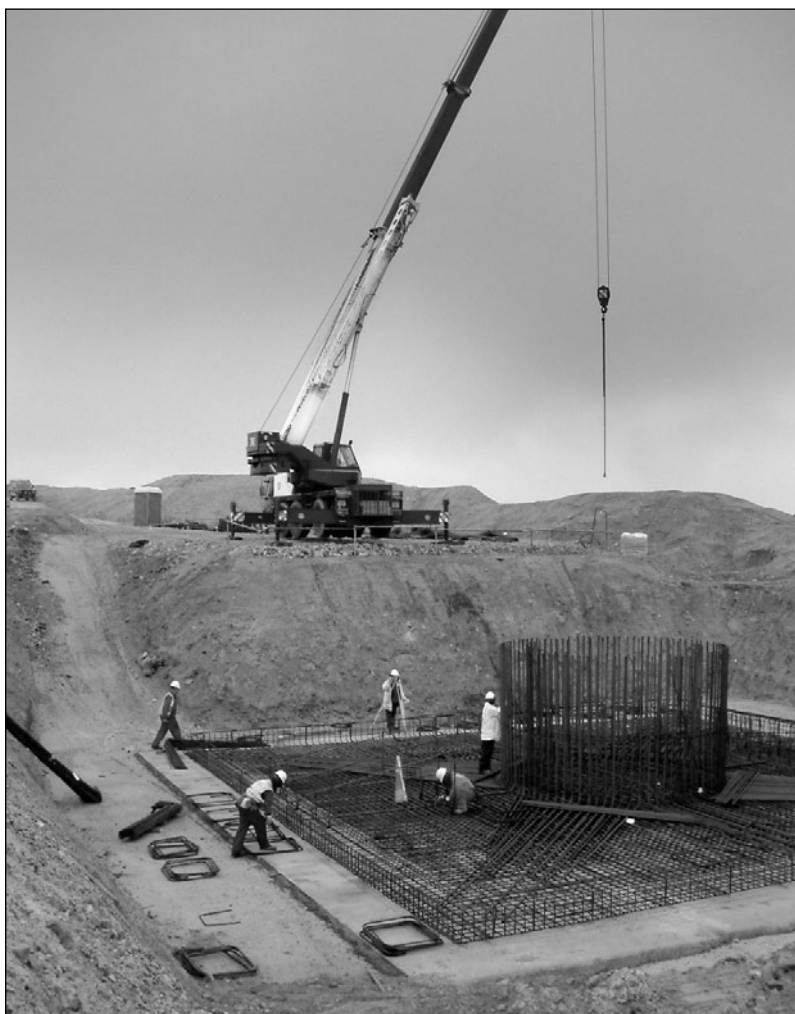
Construction of the wind farm at Paul's Hill (Bob Laughton)
