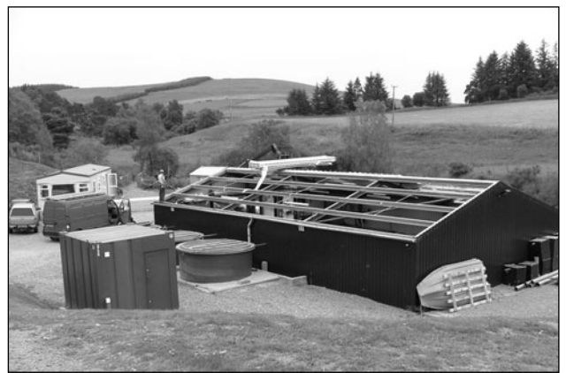
Sandbank Hatchery received a new roof in 2006 (Roger Knight)
