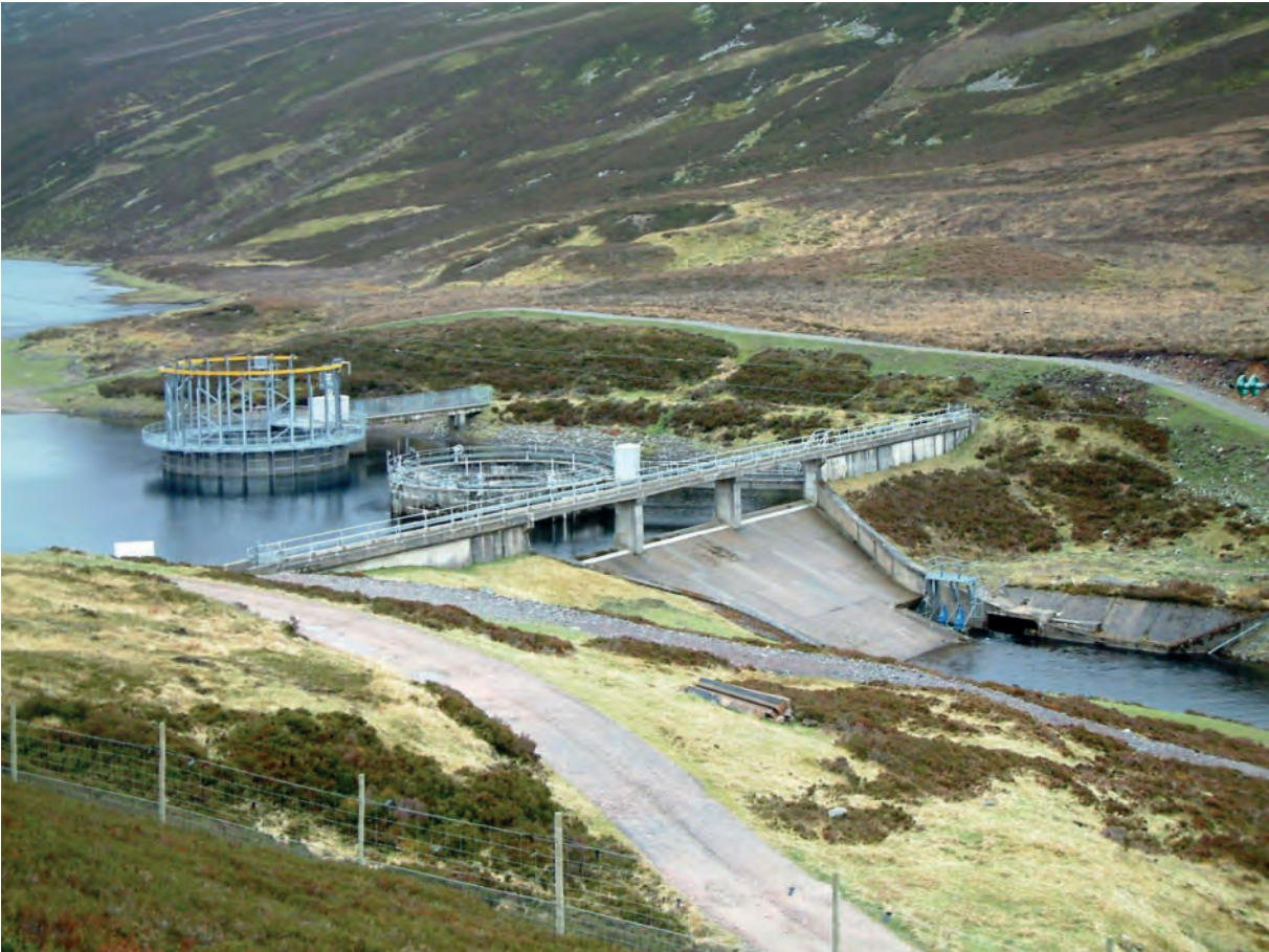
Above: Scottish & Southern Electricity’s Dam at Loch An’t Seilich on the River Tromie, from which water is diverted into the Tay catchment to generate hydro-electricity. (Photo: Dr James Butler).
