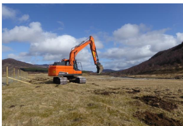
Inverted mounding in Section 1.
