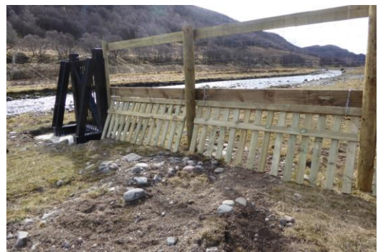
Flood plain swing fencing adjacent to water gate.
