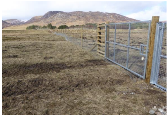
Section of deer fence showing bird strike marking and gates.
